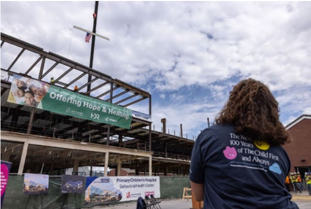
The final steel beam is placed at the new Behavioral Health Center.
